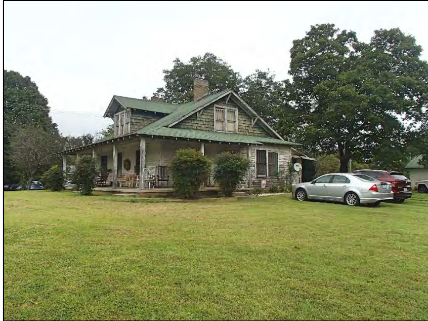
27: Frank and Maude Sowers House, southwest corner
