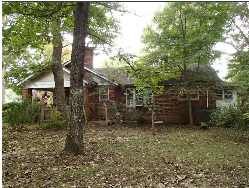
142: Shiloh Methodist Church Parsonage, north elevation
