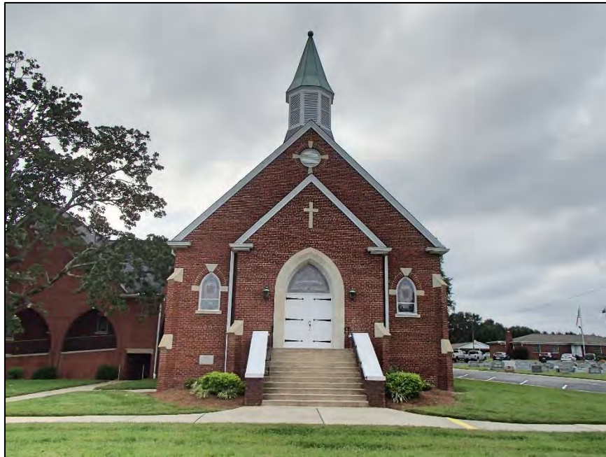
200: Good Hope Methodist Church, east elevation
