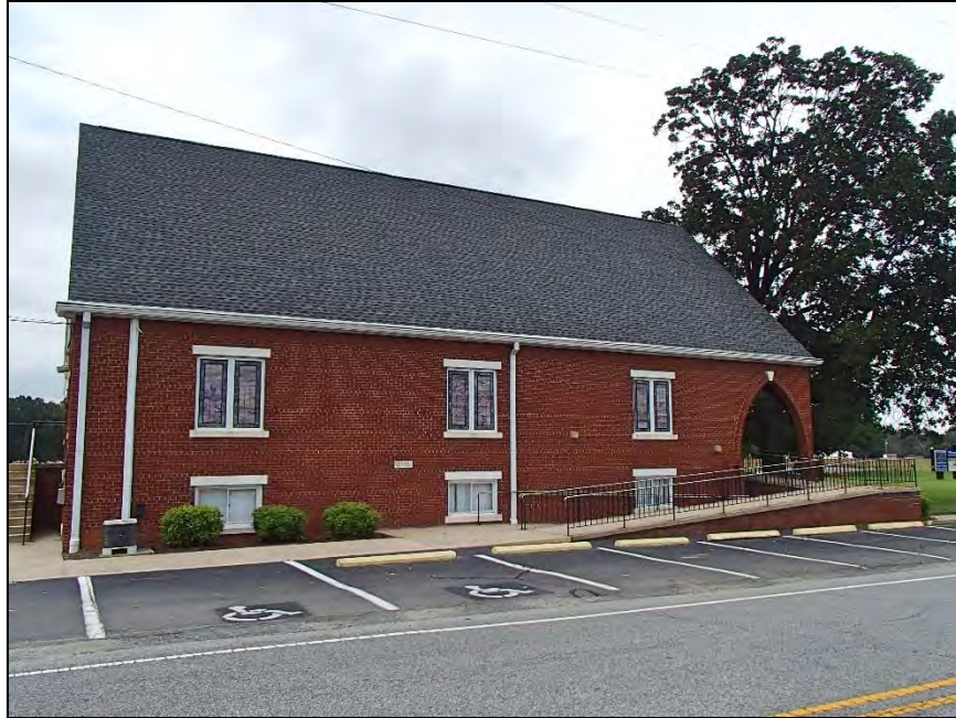
206: Good Hope Methodist Church, addition's south elevation
