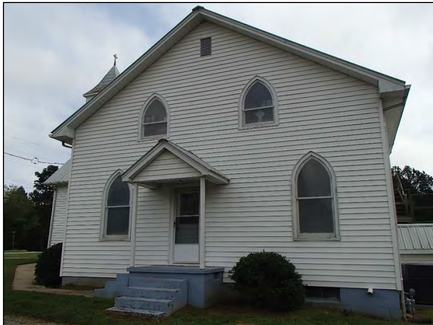
160: Maple Grove Church of the Brethren, north elevation
