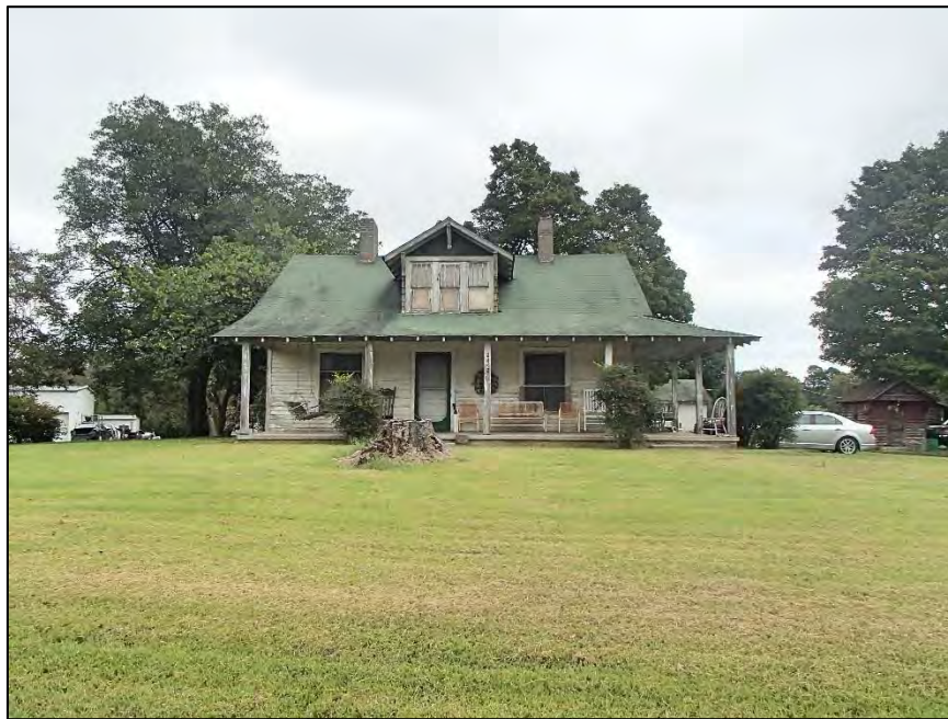
26: Frank and Maude Sowers House, west elevation
