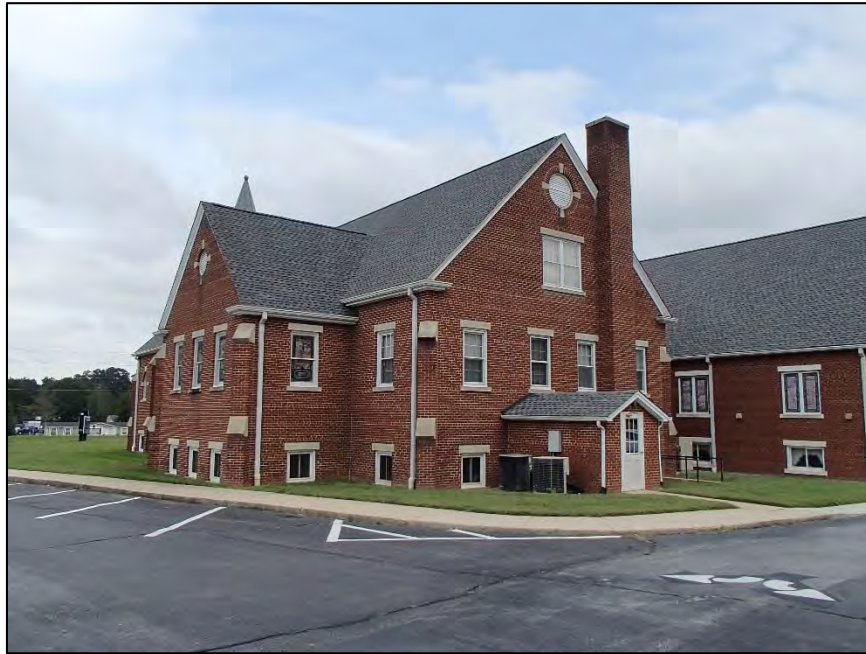
203: Good Hope Methodist Church, northwest corner
