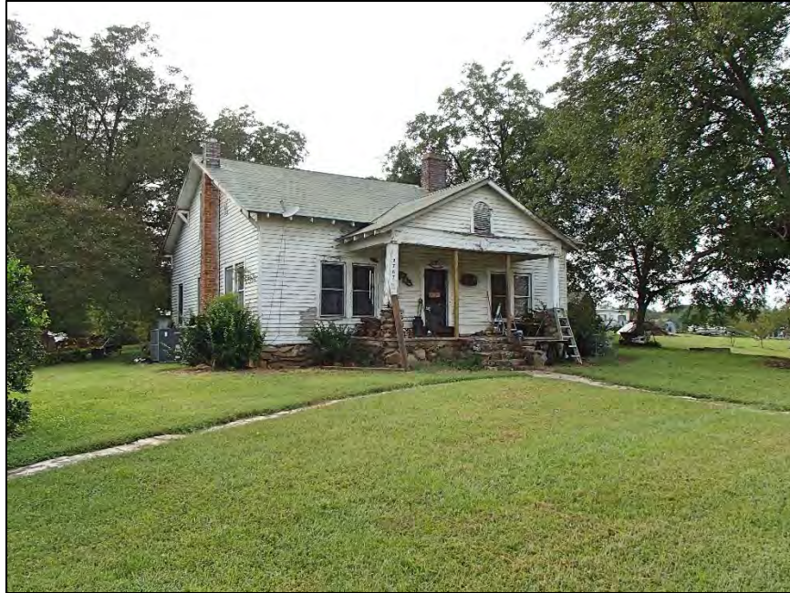
182: D.K. and Blanche Miller House, southeast corner
