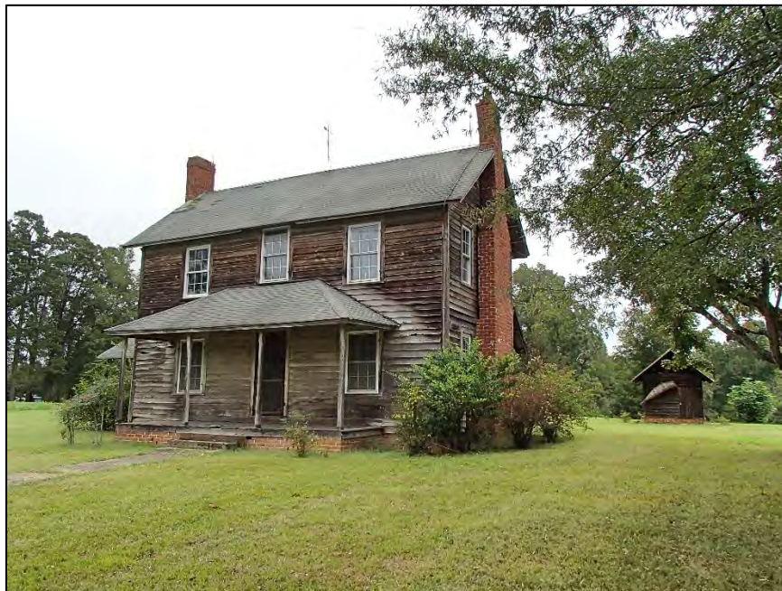
54: Felix DeLapp House, west elevation
