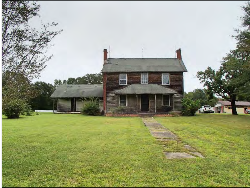
53: Felix DeLapp House, west elevation
