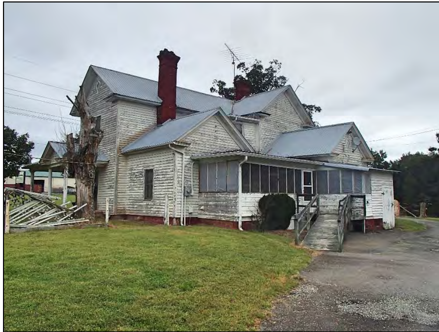
8: Lafayette and Fallie Scott House, southwest corner
