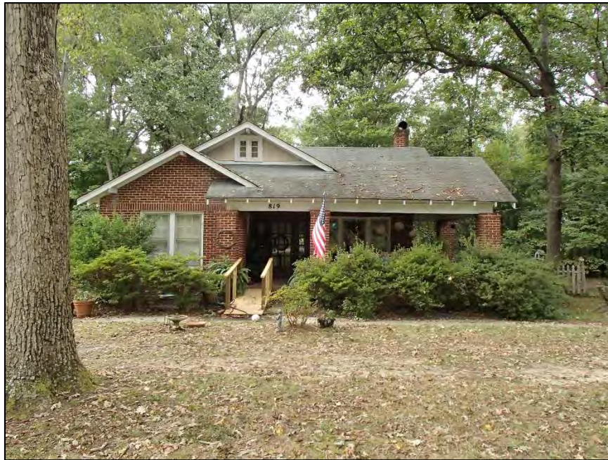
139: Shiloh Methodist Church Parsonage, east elevation
