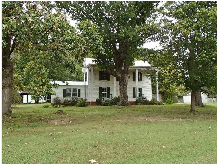
77: Unsurveyed House, showing a typical porch alteration, 515 Jake Shoaf Road
