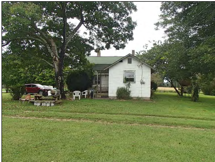
30: Frank and Maude Sowers House, east elevation
