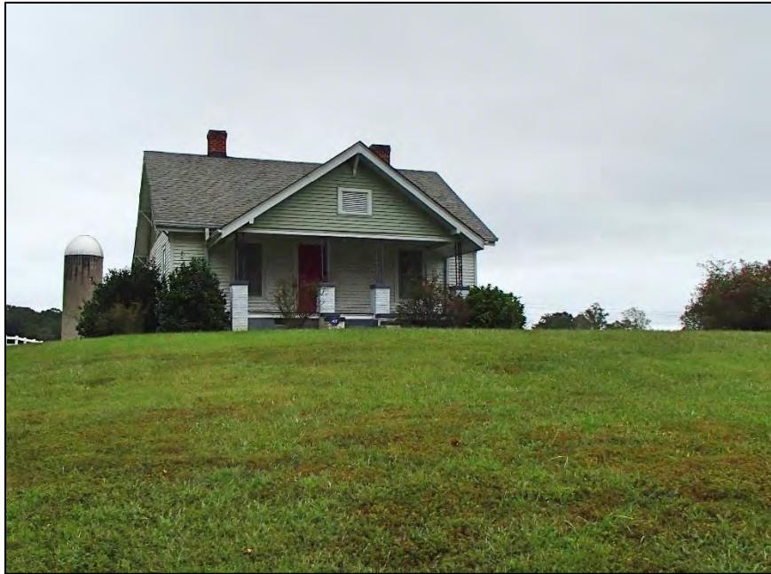
91: Unsurveyed House, Friedberg Church Road
