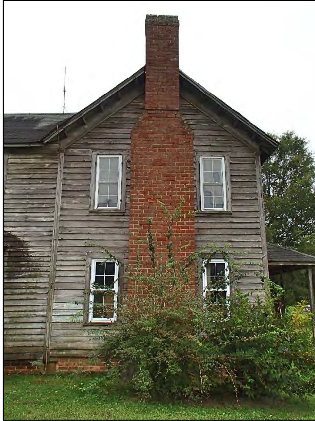
57: Felix DeLapp House, north elevation
