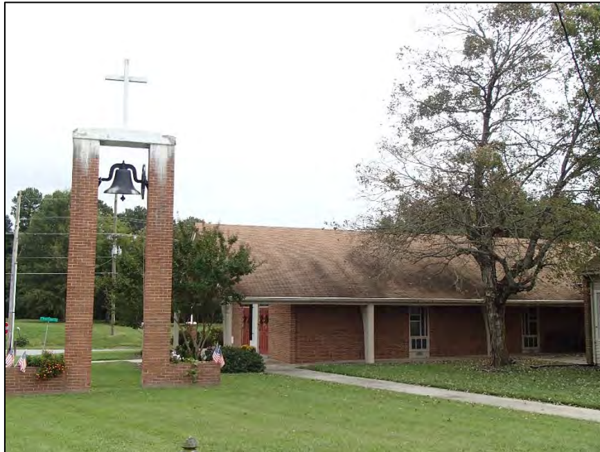
277: Arcadia Methodist Church, bell tower
