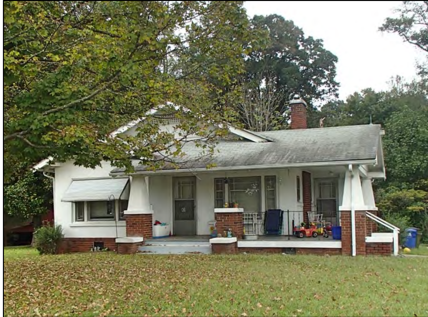
150: Unsurveyed House, stucco exterior, 1812 Hickory Tree Road
