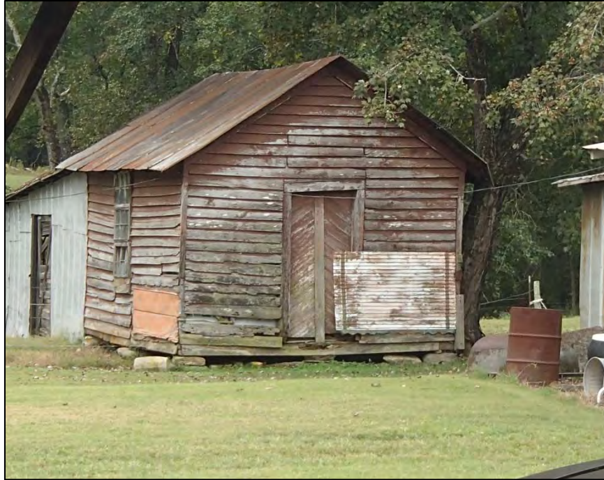
11: Lafayette and Fallie Scott House, outbuilding
