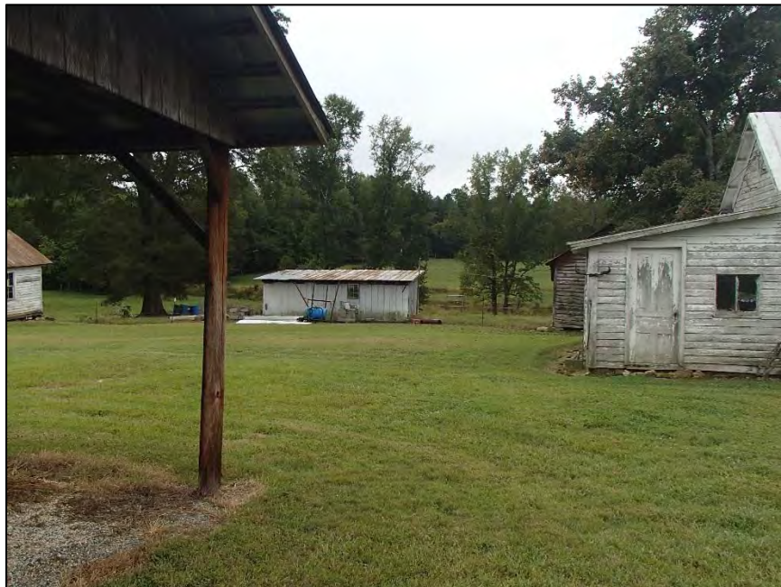
12: Lafayette and Fallie Scott House, equipment shed
