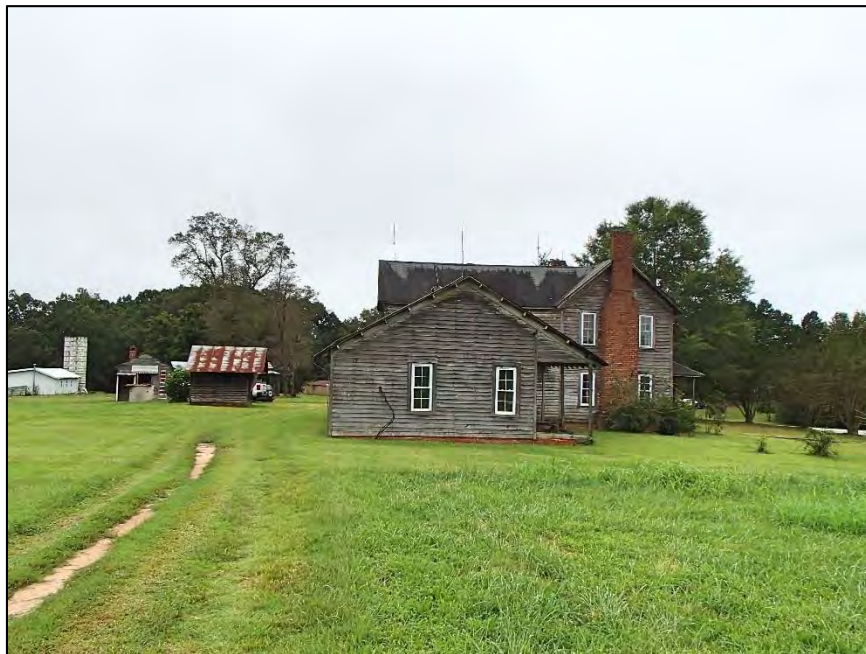
56: Felix DeLapp House, north elevation
