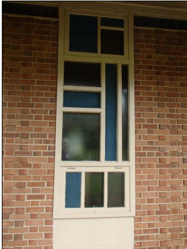
271: Arcadia Methodist Church, typical side-elevation window
