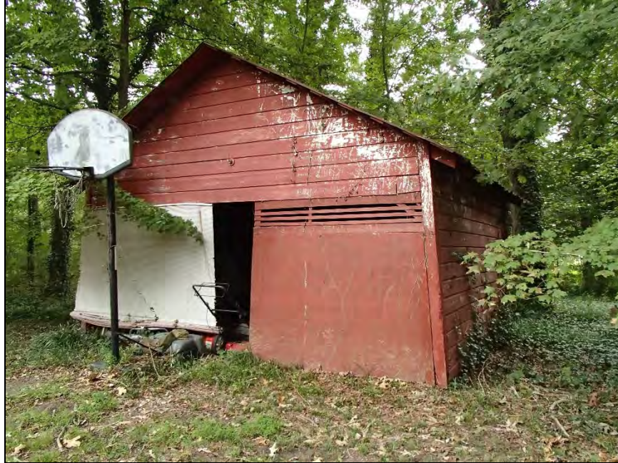
149: Shiloh Methodist Church Parsonage, garage
