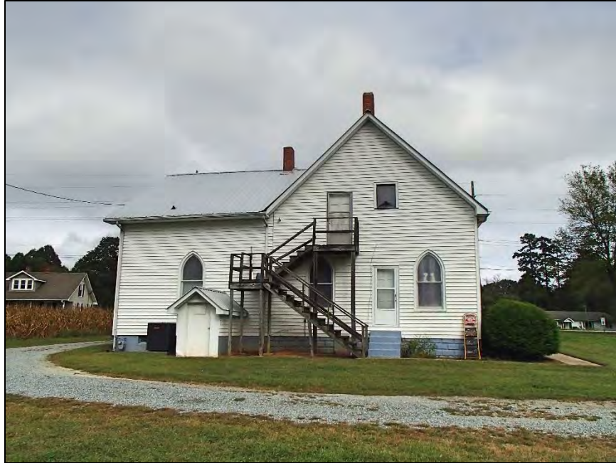
159: Maple Grove Church of the Brethren, west elevation
