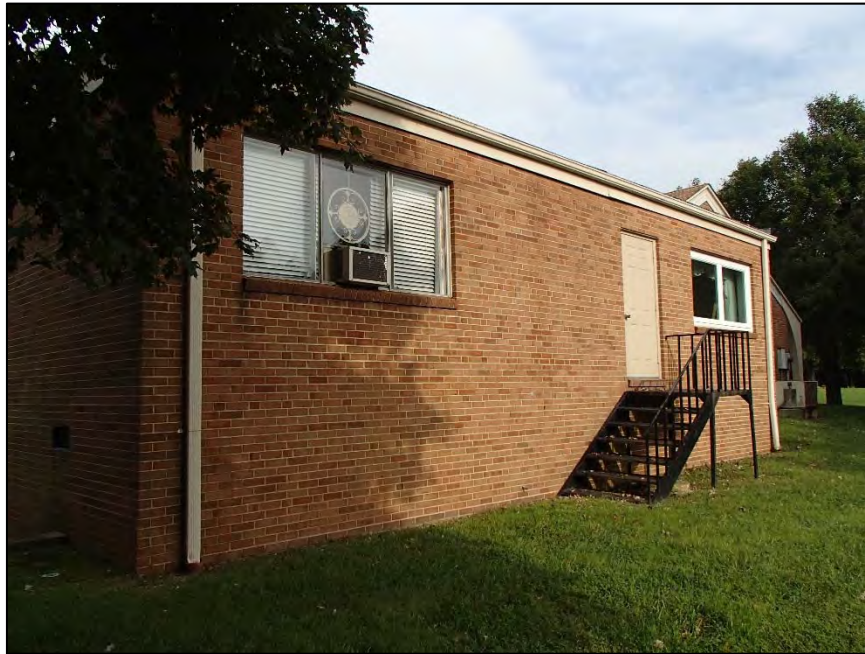
274: Arcadia Methodist Church, flat-roof addition
