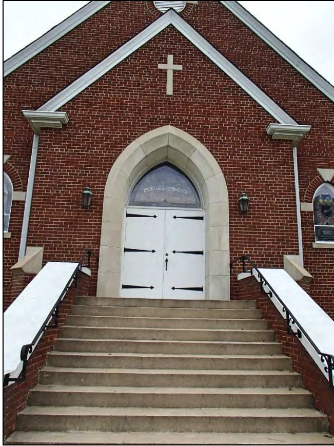
199: Good Hope Methodist Church, east elevation detail
