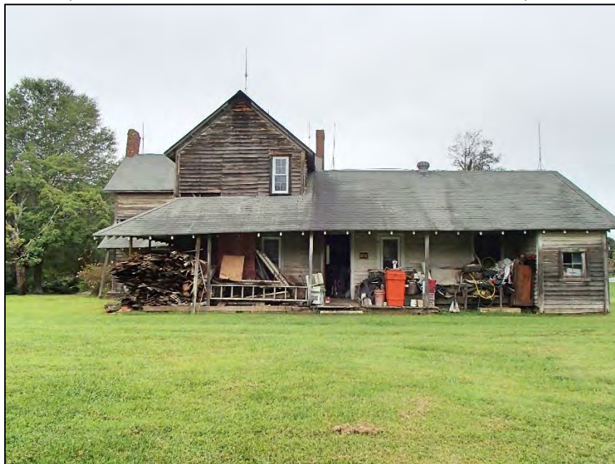
58: Felix DeLapp House, east elevation
