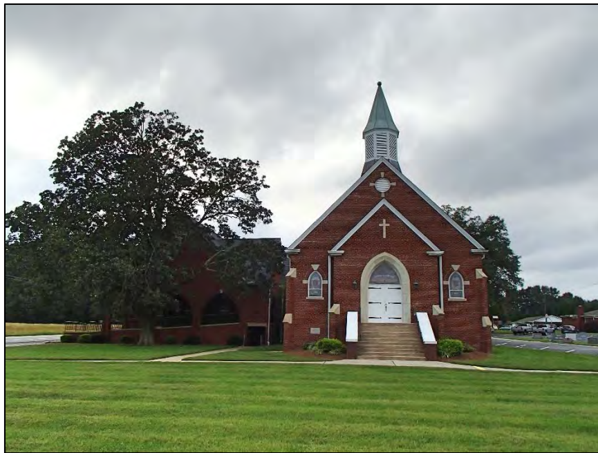
198: Good Hope Methodist Church, east elevation
