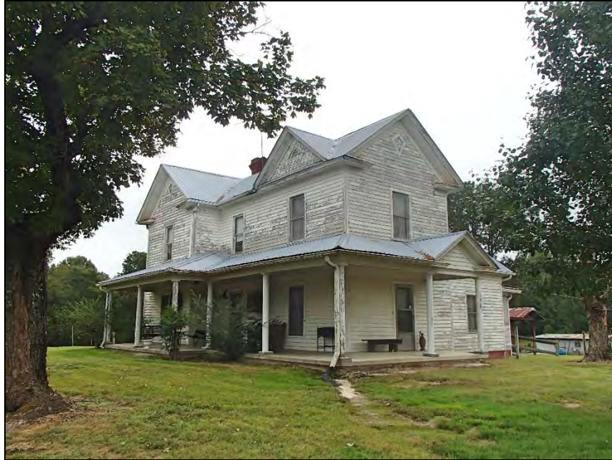
6: Lafayette and Fallie Scott House, west elevation
