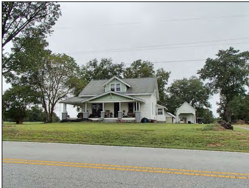
89: Unsurveyed House with well house and a barn, 9698 Hampton Road
