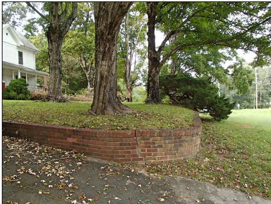
253: Manie and Letha Hege House, retaining wall
