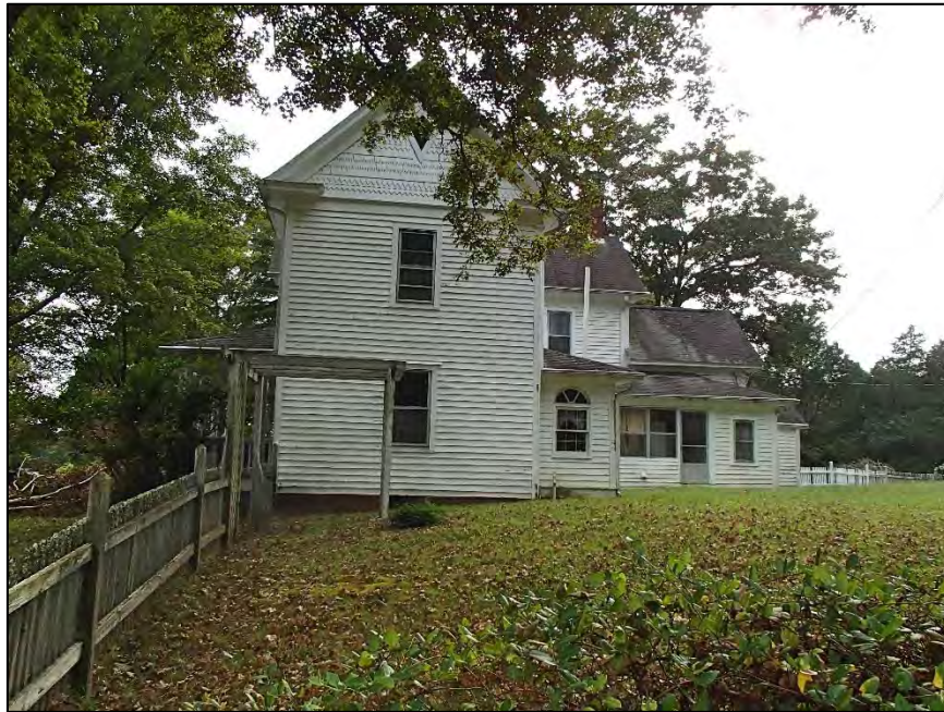
244: Manie and Letha Hege House, northeast elevation
