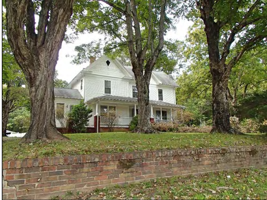
254: Manie and Letha Hege House, retaining wall
