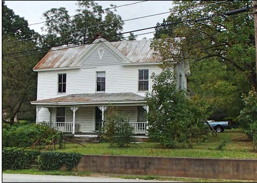
259: Unsurveyed House, 66 Bombay Road
