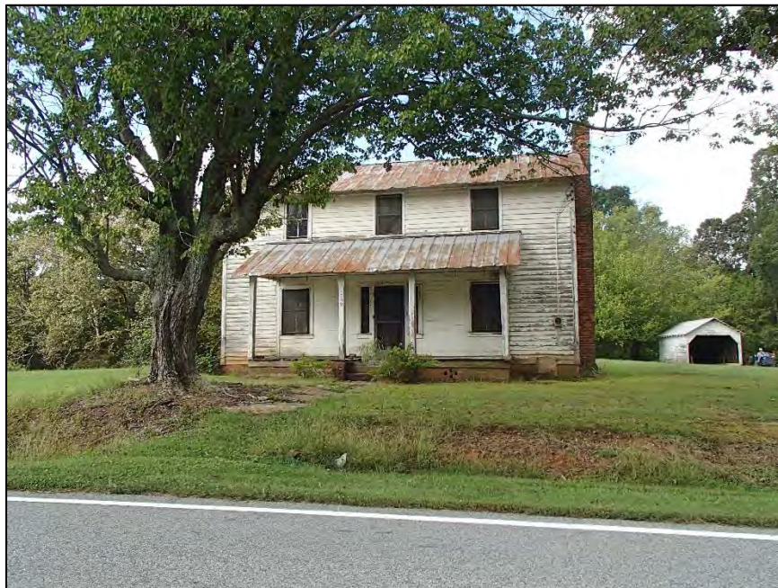
110: Old Herbert Wasler House, DV 265, Yadkin College Road; this is an I-house with chimneys on both gable ends, but the use of flushboard sheathing under the porch is similar to that at the Ollie Low Craver House
