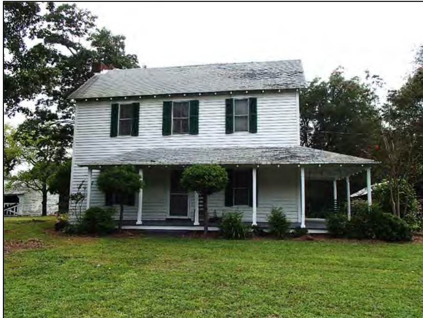
224: John D. and Addie Hill House, east elevation
