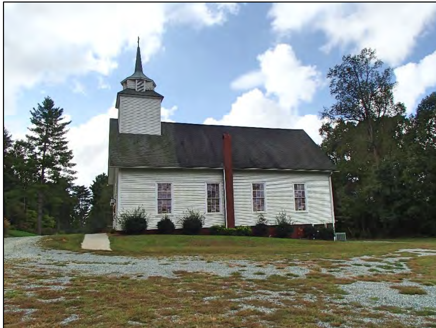
174: Yadkin College Methodist Church, DV 58, NR-Listed in the Yadkin College Historic District
