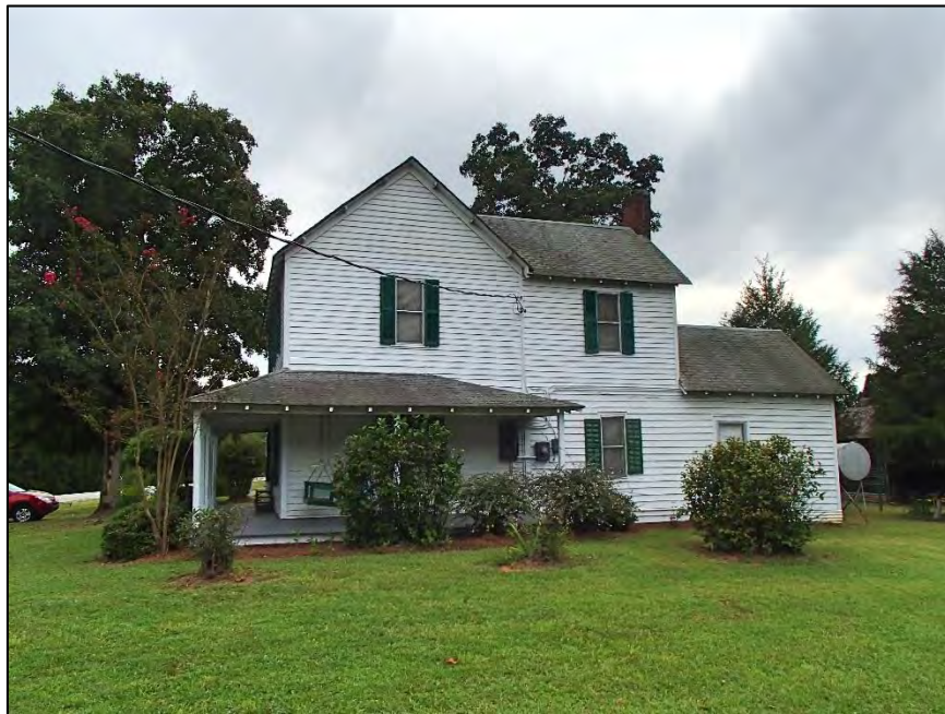
226: John D. and Addie Hill House, north elevation
