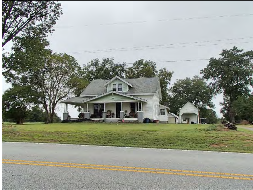
127: Unsurveyed House with well house and a barn, 9698 Hampton Road
