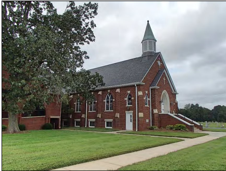
201: Good Hope Methodist Church, southeast corner
